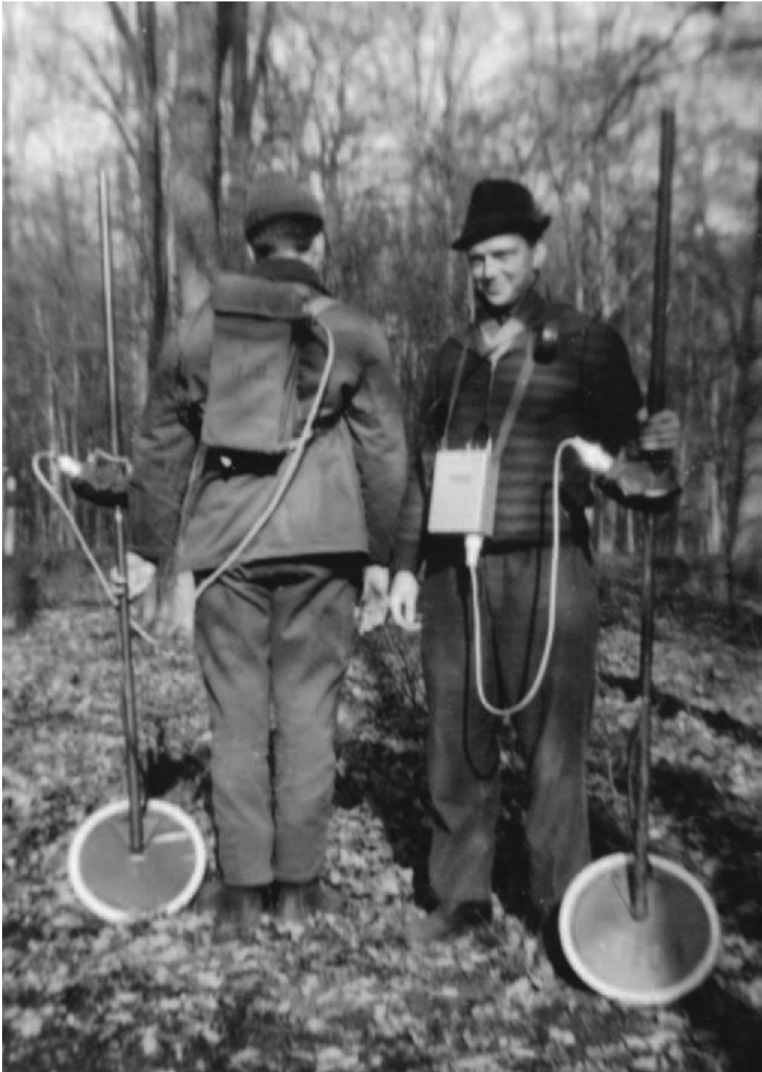
Fig. 9 SCR 625 in the original and in transistorised version
